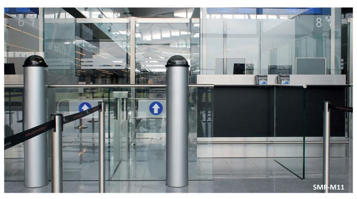
**SMP-M11** or **SMP-M22** Radiation Portal Monitors (RPMs) are equipped with one or two measuring columns, respectively, to perform functions of detection and preliminary processing of the signals, and a control panel with a touch screen and printer.
